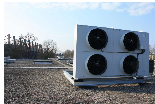
Free-Cooling (air indirect)
